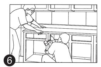
Place your counter top into position and make sure it is held tightly against the wall to ensure the best fit (use 3/4" thick 1x2's to raise the counter top to the correct height). Then anchor the counter to the cabinets using the corner braces provided on each cabinet. Be careful not to screw too far or use screws that are too long because you may damage the counter top.
