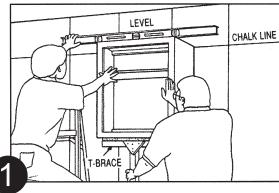
Make a T-brace tall enough to support a wall cabinet at the height that you marked on the wall. While you and a helper steady the cabinet on the top of the T-brace, level it and check that the top stays even with your guideline.
