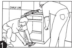
Starting at the highest point on the floor; place the first cabinet into position according to your plan. Use your level to see if your cabinet is both level and plumb. If it is not, use shims on the floor to bring the cabinet plumb. A wooden block can be used to used to avoid damage to the floor or wall when driving shims.
